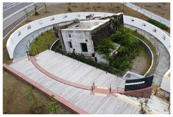
The former Onagawa Police Box is a two-story reinforced-concrete building whose foundation was ripped out of the ground by the receding tsunami wave produced by the Greart East Japan Earthquake. It is one of the rare cases in the world where a reinforced-concrete building collapsed or was topped over by a tsunami.
